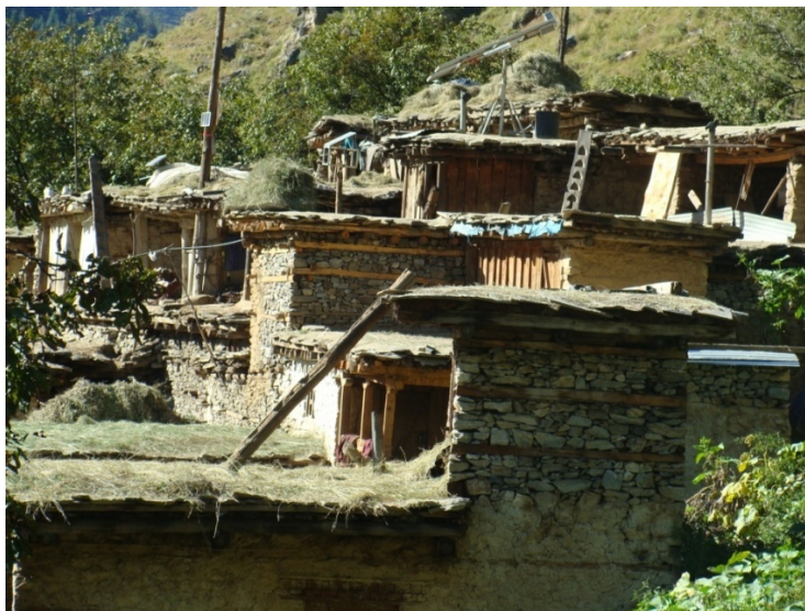
Figure 4. Typical Cluster System. Note the photovoltaic panel in the top center. It is connected to a battery bank servicing six households in this section of the village.
