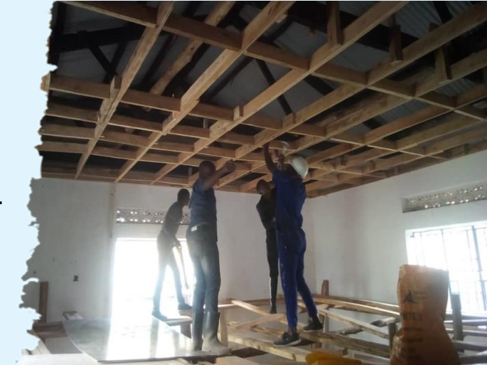
Renovations at the Nakaseke SCBU
