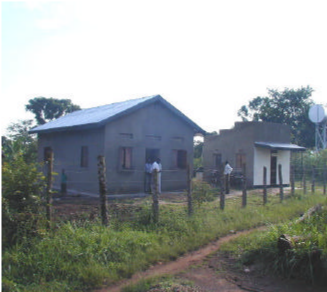
Plate 13: The ISISfunded Community Based Health Care Hall.
